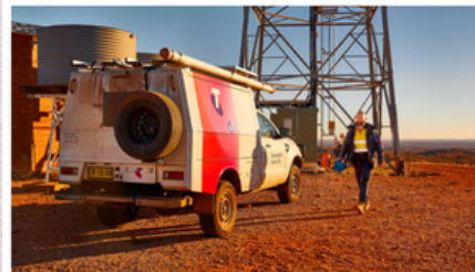
To upgrade mobile towers to 4G and 5G technology, they need to be switched off for safety reasons. (Supplied: Telstra)
